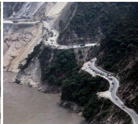
Fig.2(b)Damage of Roads (CBIP,2013)
