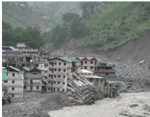
Fig.2 (a): Destruction of Buildings
