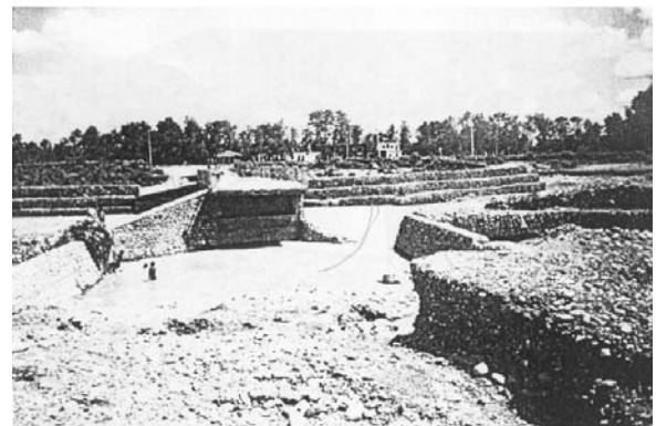
Fig. 8 Outflanking of bridge on river Danabkhola in Nepal
