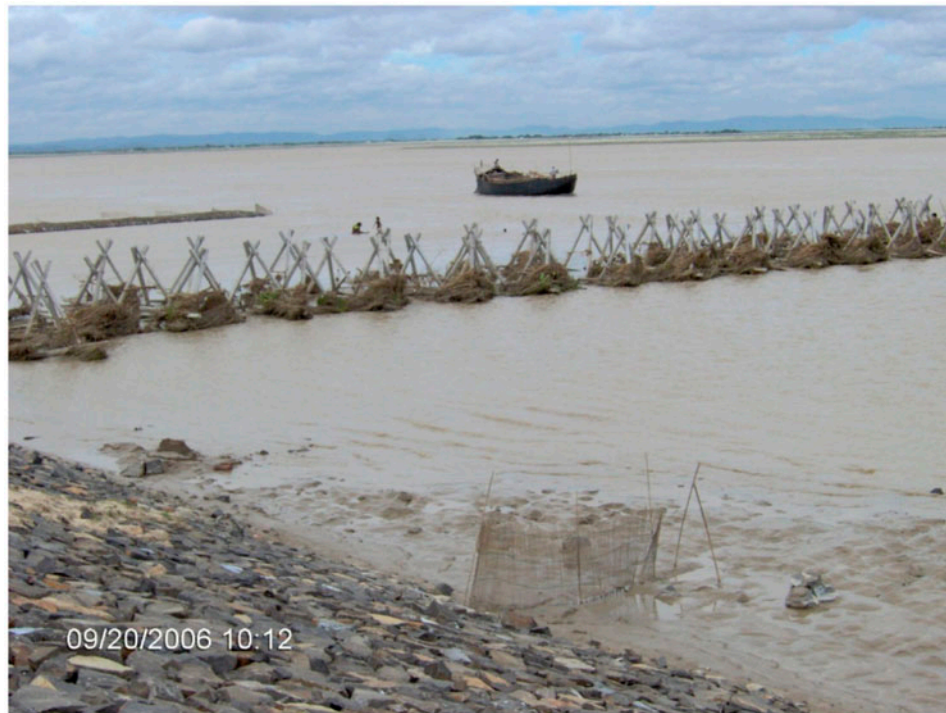
Figure 1. Showing one row of RCC porcupines used upstream of the Farakka Barrage.
