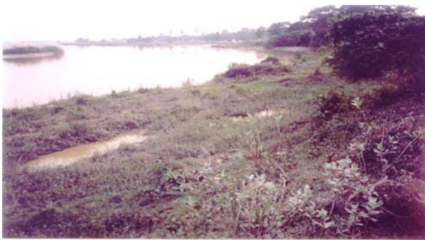
Fig. 16 Erosion on left bank of Bagmati River eroding the habitats U/S of bridge
