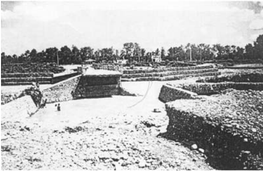
Fig. 9 Outflanking of a vented causeways on the stream 'Danab Khola' in Nepal
