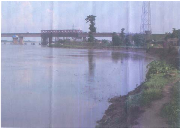
Fig. 12 Erosion on Right Bank of Mahananda River Showing Embayment U/S of the Bridge
