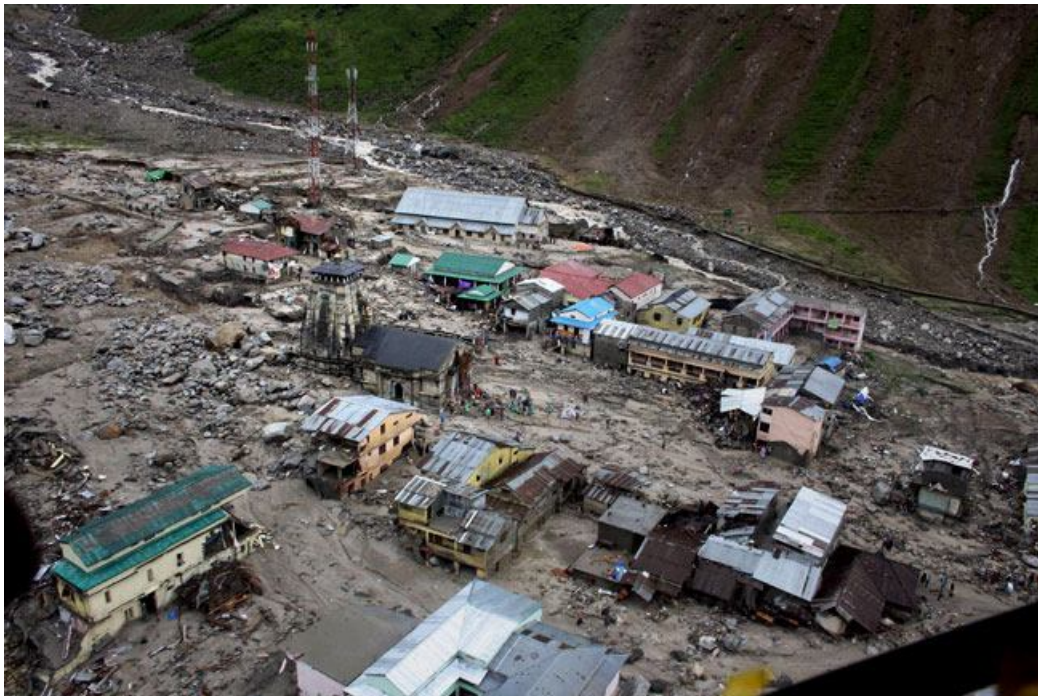
Fig.11 A view of the washed off buildings in Kedarnath Dham in Uttarakhand following incessant rains and floods. (PTI photo). Kedarnath Temple can be seen in the photograph.
