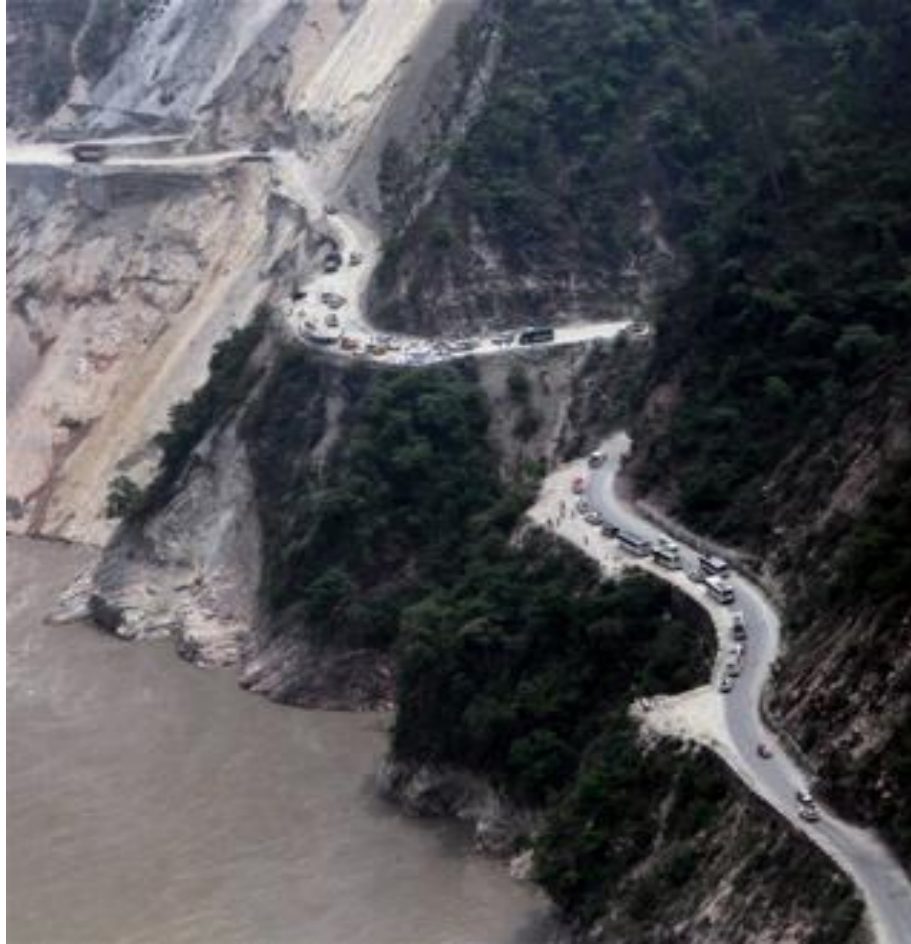
Photo-3 Typical road damage by landslip in Srinagar, Uttarakhand.
