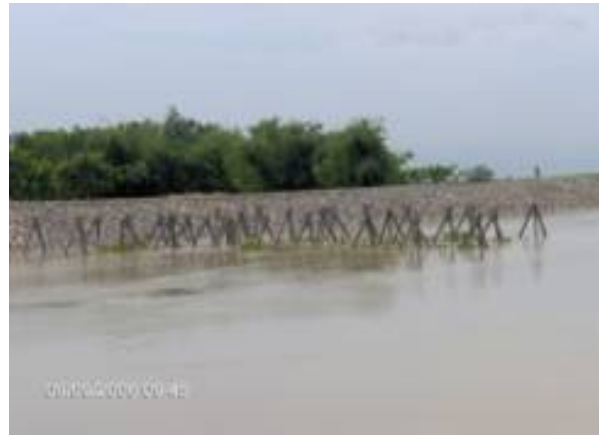
Fig.11 Porcupines used for Protection Left Embankment Spur in Farakka Barrage
