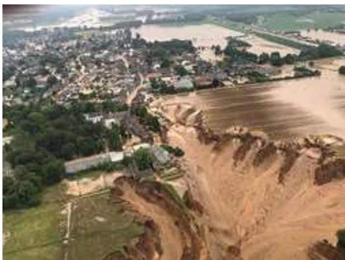
Photo-3: Showing flooding in Erfstadt Germany. Rhein-Erft District in July 2021
