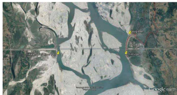
Fig.6: Bogibeel Bridge (4.9km long) on Braided Flood Plain of River Brahmaputra
