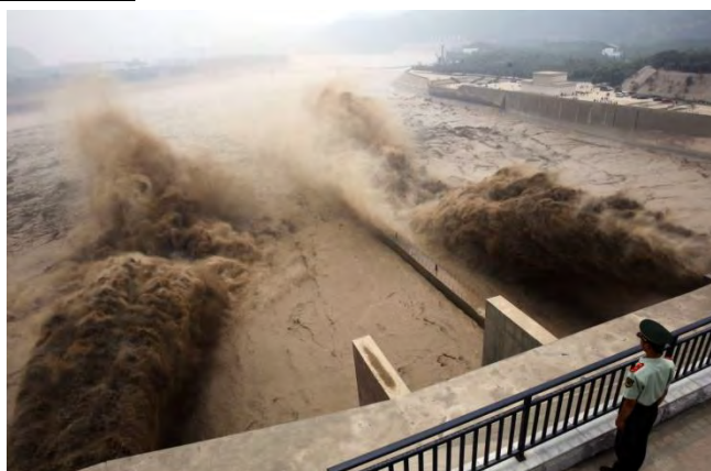
Fig. 11 Sediment Flushing from Xiaolangdi Dam on Yellow River in China
