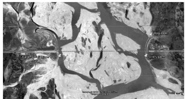
Fig. 8 (b) Bogibeel Bridge on Braided River Brahmaputra
