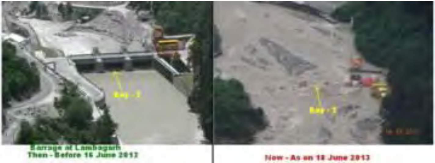
Fig.1 Aggradation Due To Landslides in 2013 Flood in Uttarakhand
